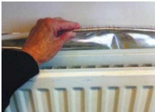
It's easy and cheap to put reflector foil behind radiators fixed to outside wall. The foil makes sure you just heat your house, and not the rest of Oxfordshire.
